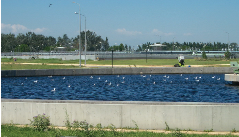
Figure 3-48 Primary sedimentation tanks in Thessaloniki's WWTP
