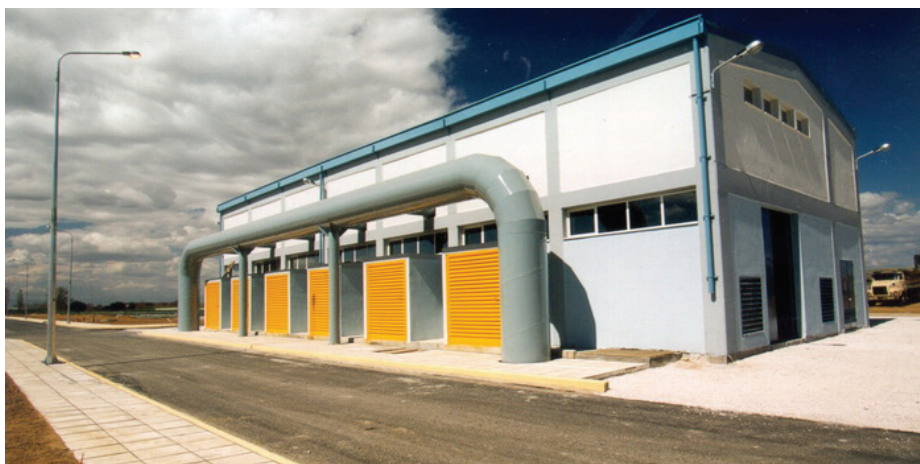
Figure 3-51 Thessaloniki's WWTP is equipped with 5 aeration units
