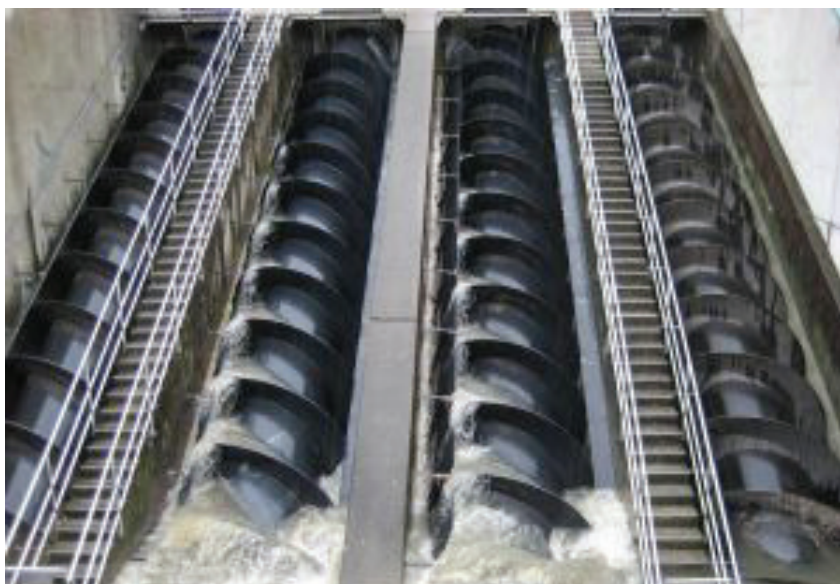
Figure 3-49 Archimedes screw pumps
