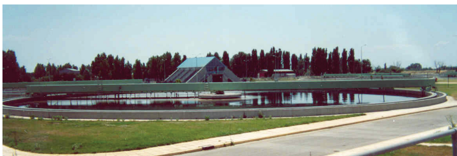
Figure 3-52 Final sedimentation tanks at the WWTP of Thessaloniki
