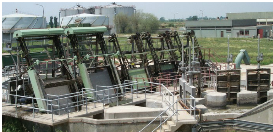
Figure 3-46 Bar screens (5 lines) at Thessaloniki's WWTP
