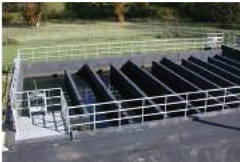
Figure 3-53 Disinfection of treated wastewater with chlorination
