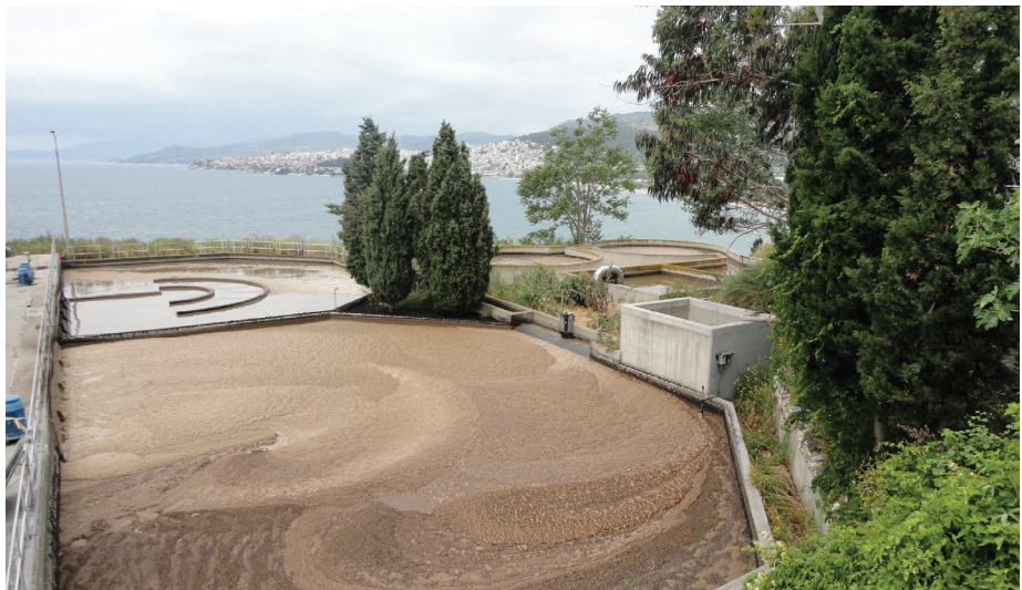
Figure 3-10 Phosphorus removal before the biological treatment in Kavala’s WWTP
